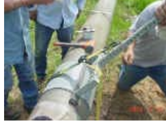
Step 3 - Tighten the Sleeve
