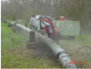
Step 1 - Prepare the Pipe Surface
