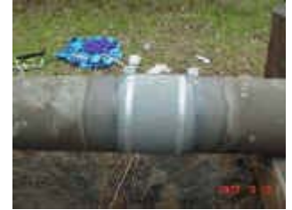
Step 4 - Completed Installation
