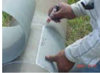
Step 2 - Mark and Apply the Sleeve
